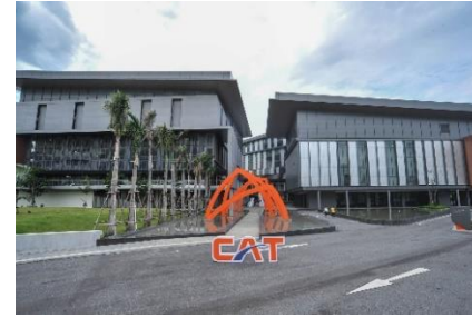
CAT Telecom 21 units
